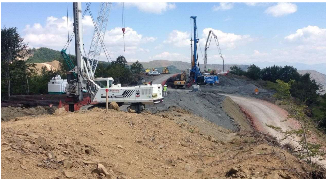
Fig.2 Works during TAP Project in Vithkuq
