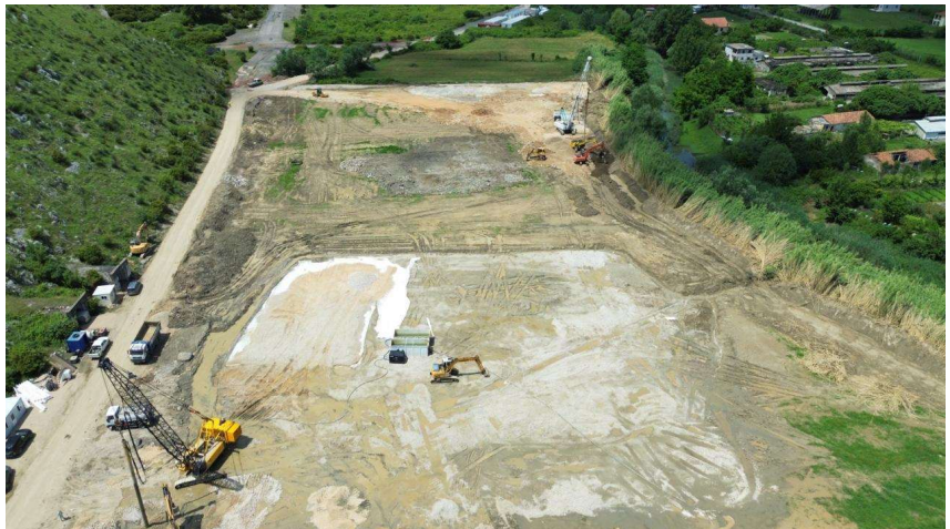
Works during construction of top feed stone columns for Gjader Project
