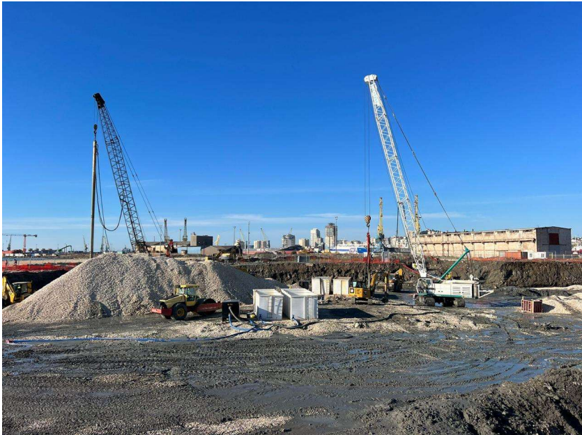
Works during construction of top feed stone columns for Durres Yacht and Marina project
