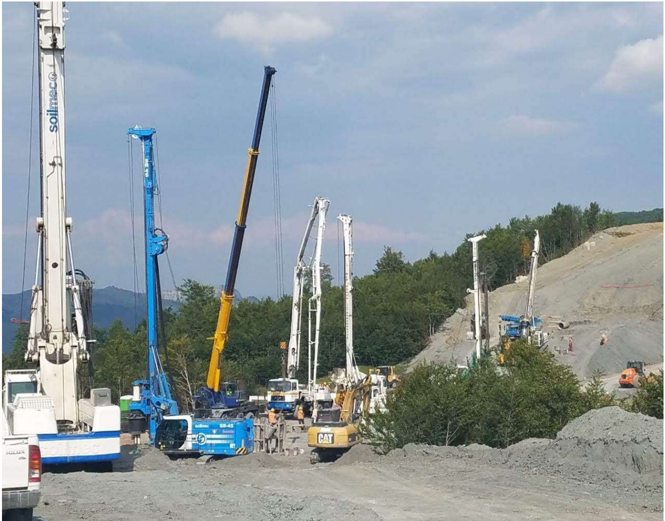
Fig.1 Works during TAP Project in Vithkuq
