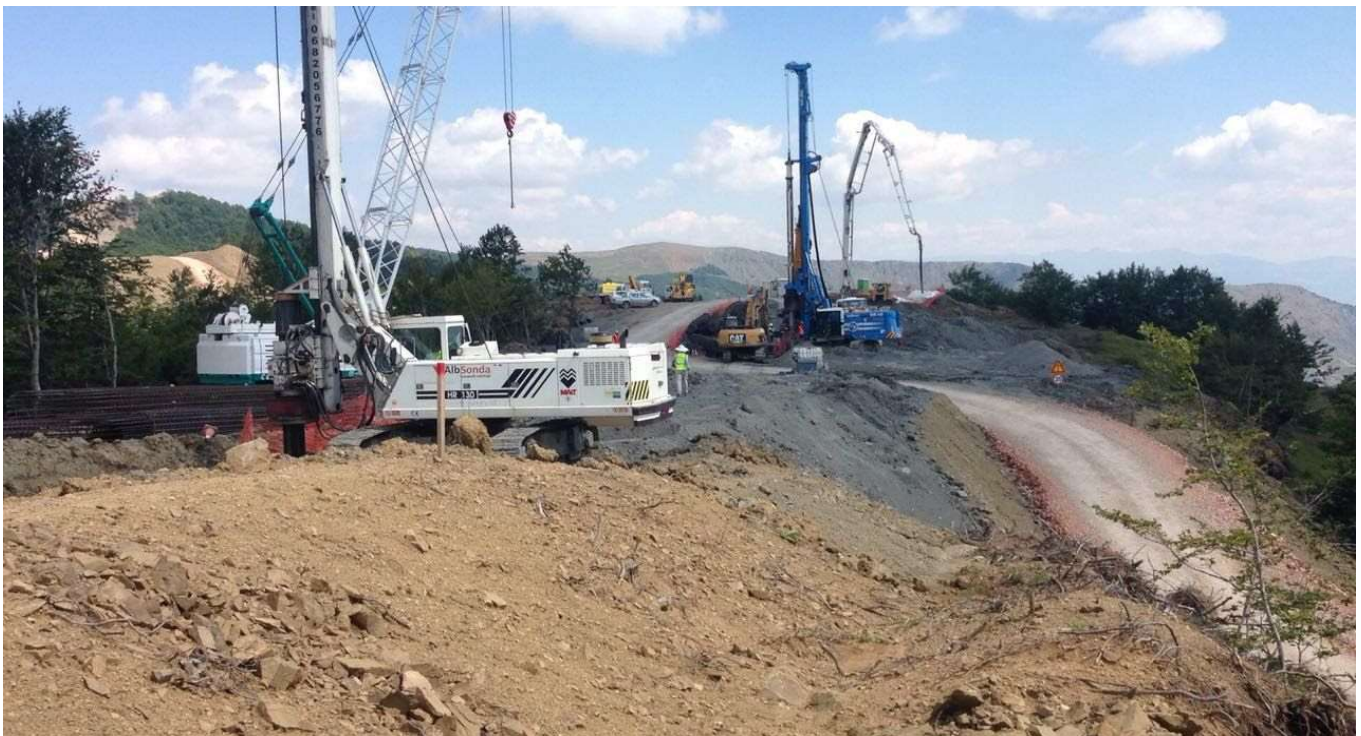
Fig.2 Works during TAP Project in Vithkuq
