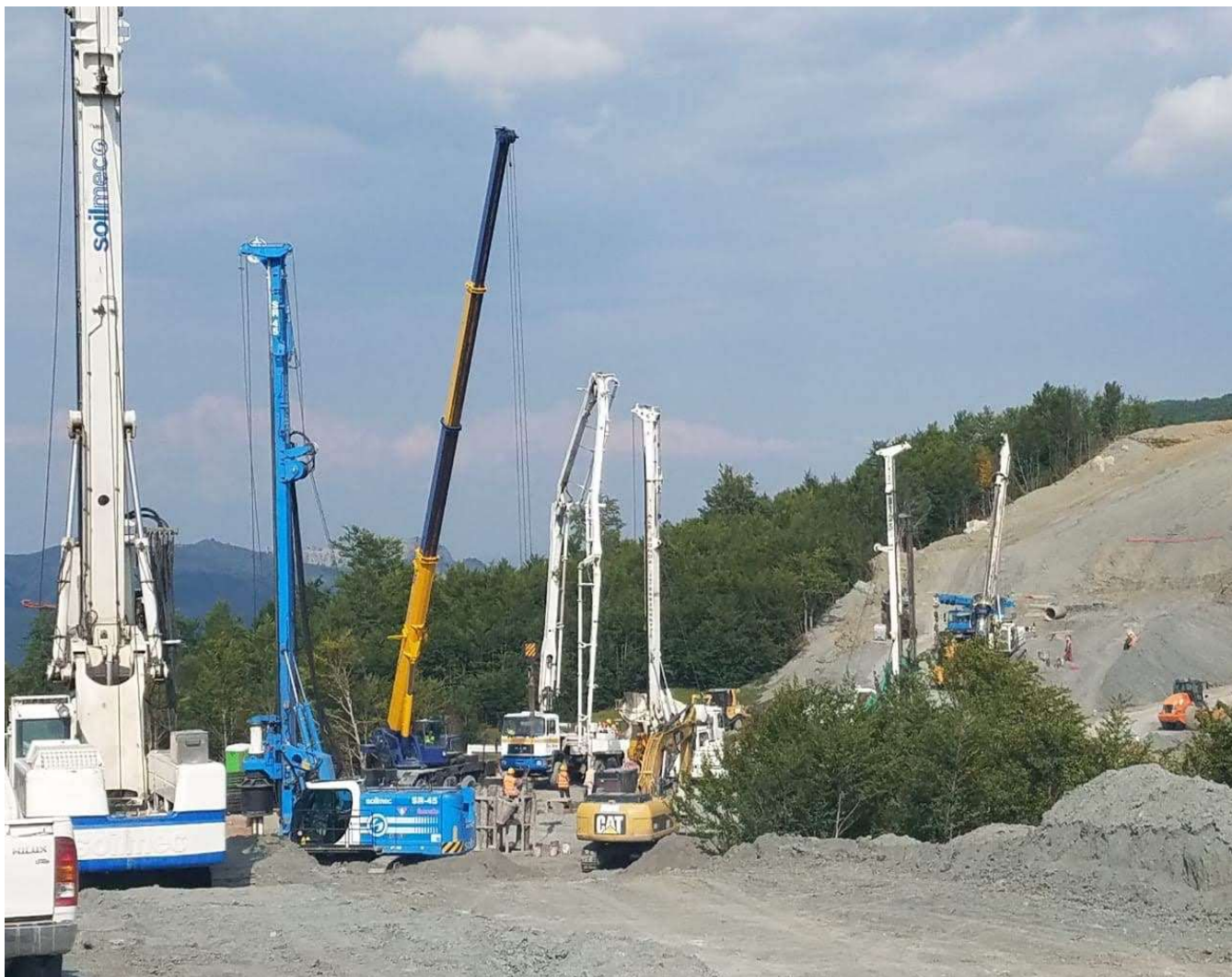
Fig.1 Works during TAP Project in Vithkuq
